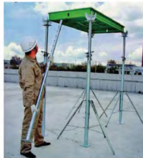
Put the other props in position
