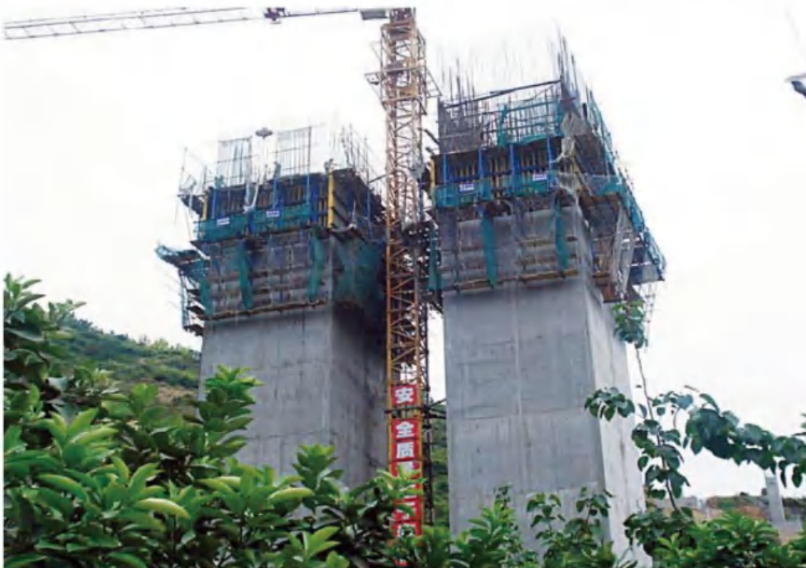
Yalu Expressway Bridge, Sichuan, China
