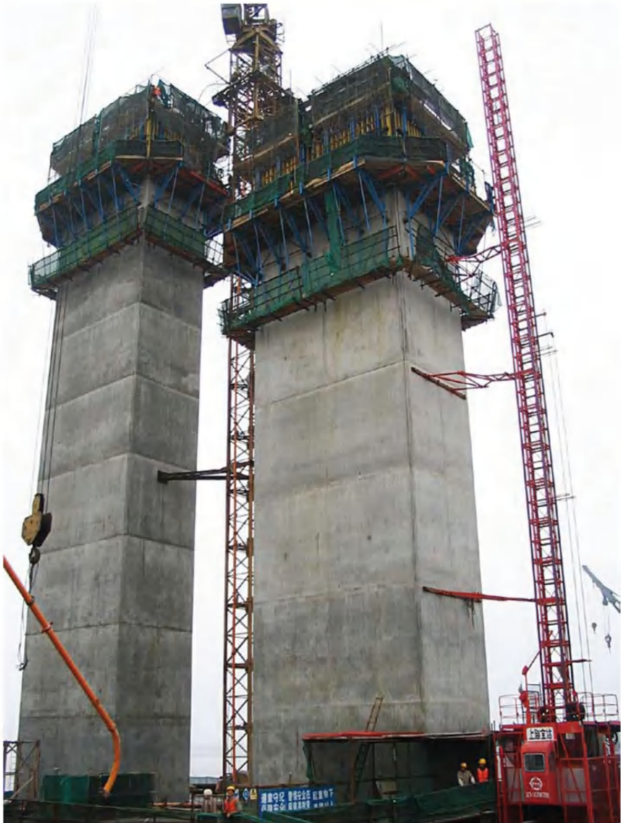
Sutong Bridge, Jiangsu, China
