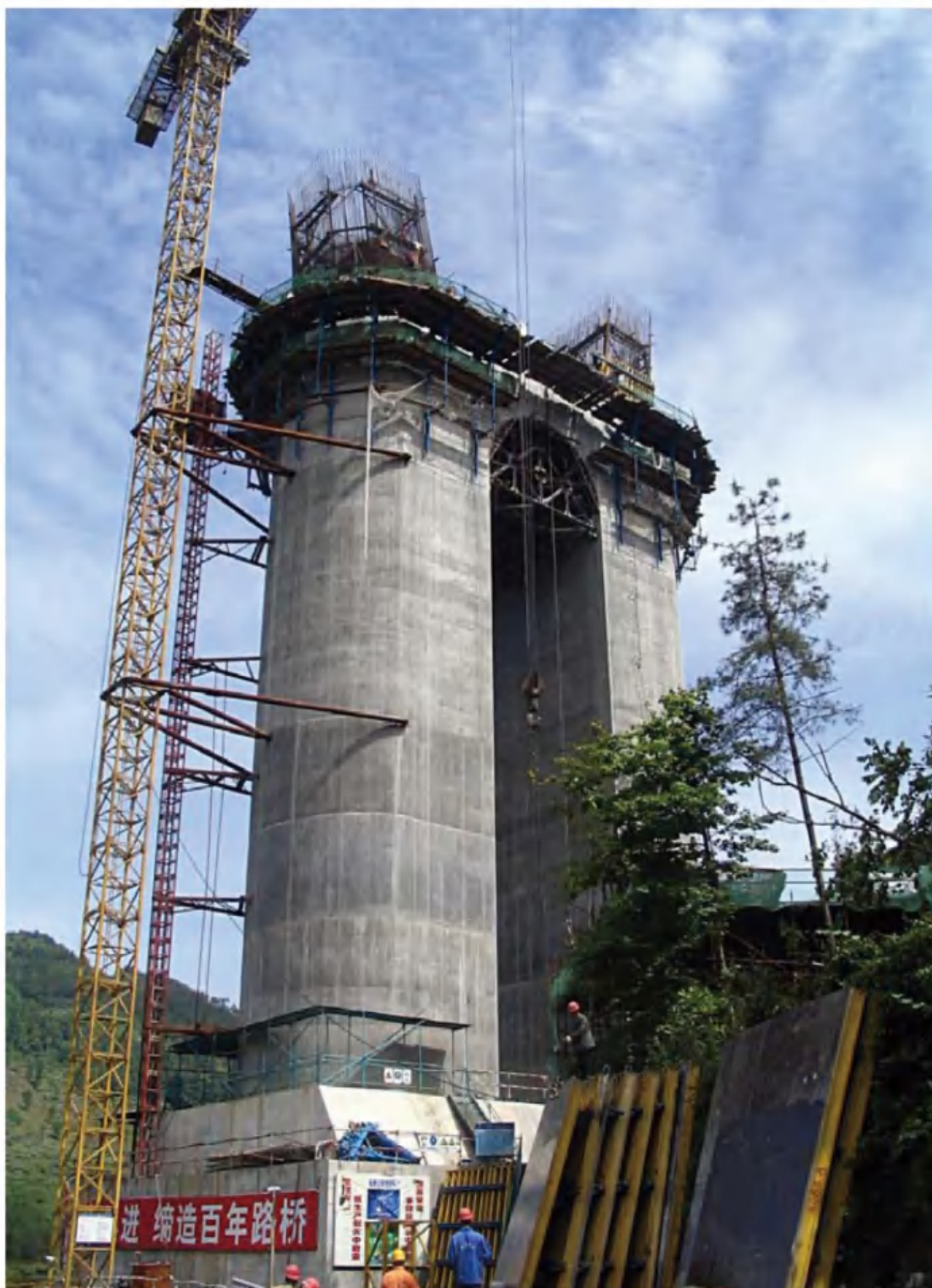
Ganxigou Bridge, China
