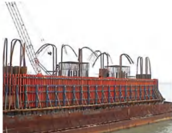
The Forth Qianjiang Bridge, Zhejiang, China
