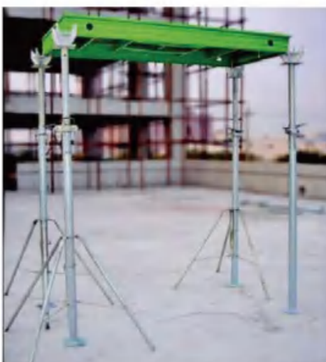
Check the elevation of formwork
