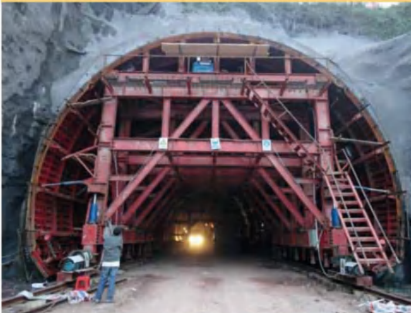
Project: Datong—Xi'an high railway User: China Railway 2nd Bureau Technical Data: length 9m; radii 6.7m; weight of trolley 81.5t Site photograph
