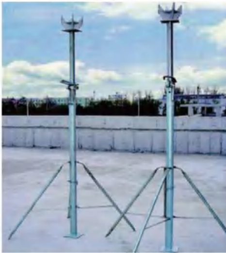
Set up the prop and tripod system
