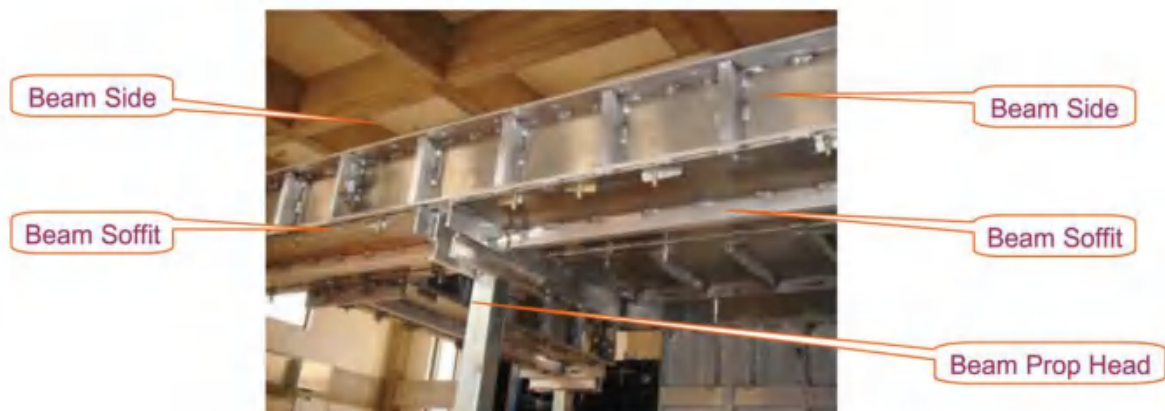
The Use of the Beam Prop Head
