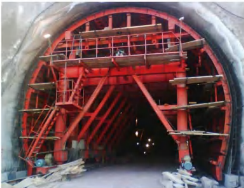
Project: Jinzhou—Chifeng railway User: China Hydropower 14nd Bureau Technical Data: length 12m; radii 2.5m; weight of trolley 70t Site photograph
