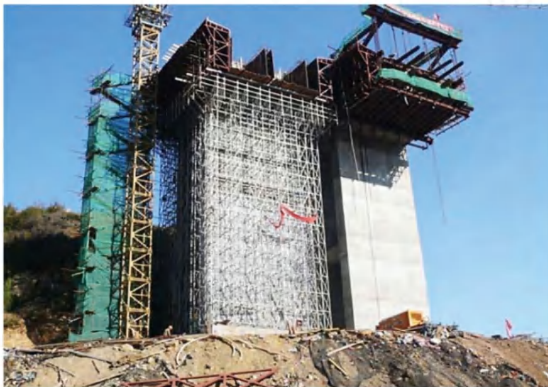
Highway Bridge, Guizhou, China
