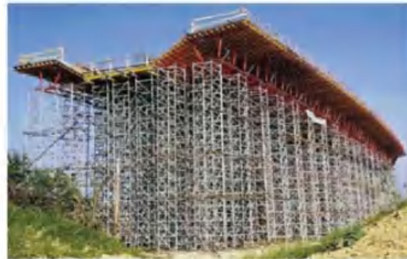
Girder Box Formwork
