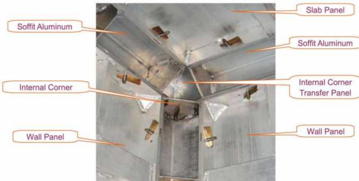
The Connection of Slab Panel, Wall Panel, Internal Corner panels and Soffit Aluminum
