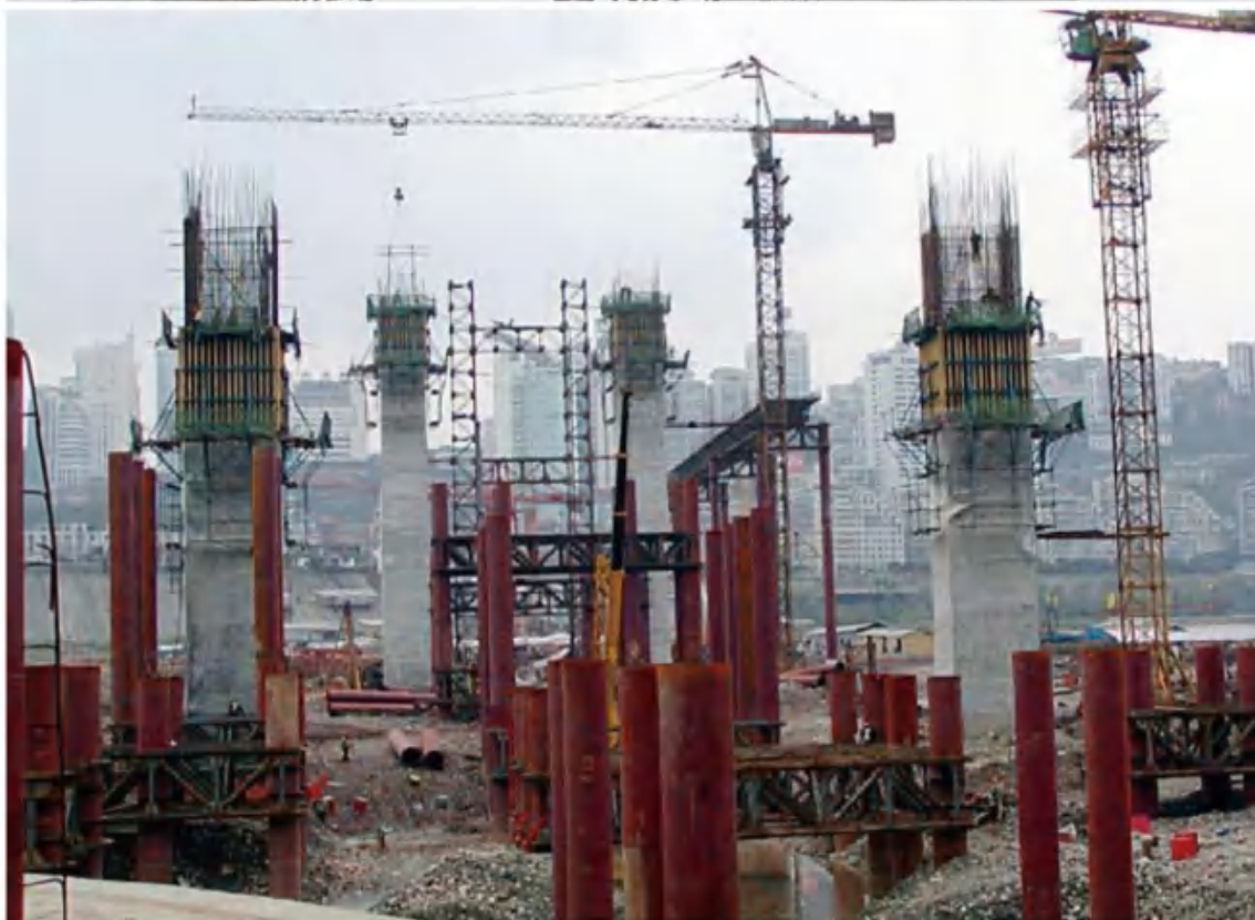
Xiarong Express Way Bridge, Guizhou, China
