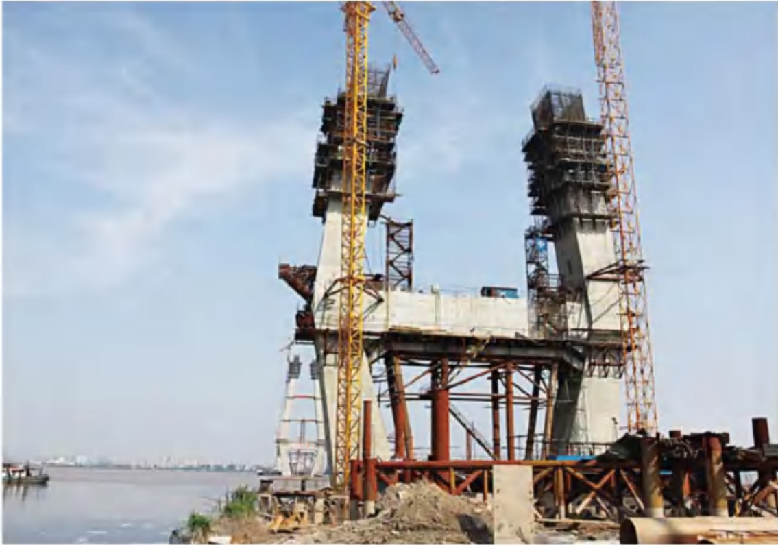
Tinxingzhou Bridge, China
