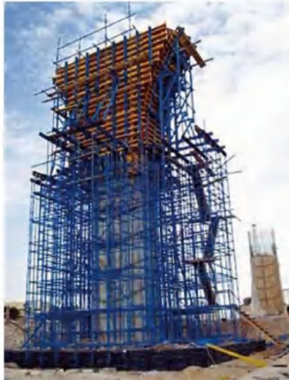
Style Design Formwork
