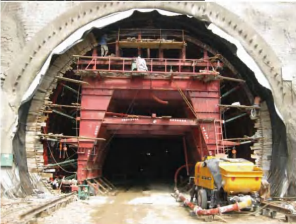
Project: Beijing City Railway User: China Railway 21nd Bureau Technical Data: length 12m; radii 6.7m; weight of trolley 115t Site photograph
