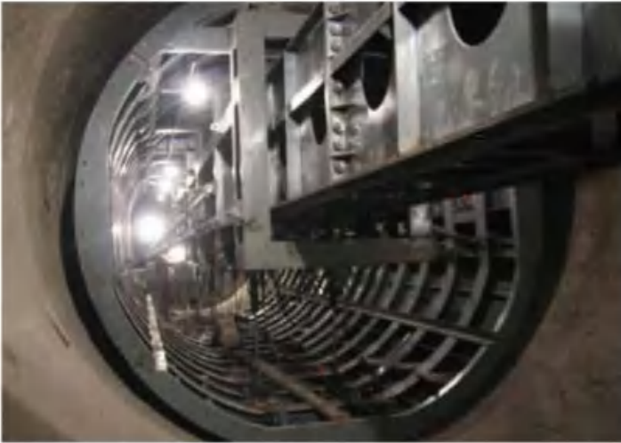
Project: Xinjiang Water Channel User: China Railway 11nd Bureau Technical Data: length 12m; radii 1.85m; weight of trolley 46t Site photograph
