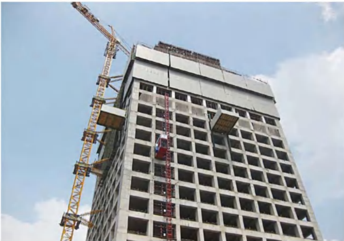
Service Platform for Science and Technology, Harbin, China
