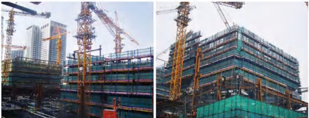
Jing-ao Commercial Building, Beijing, China
