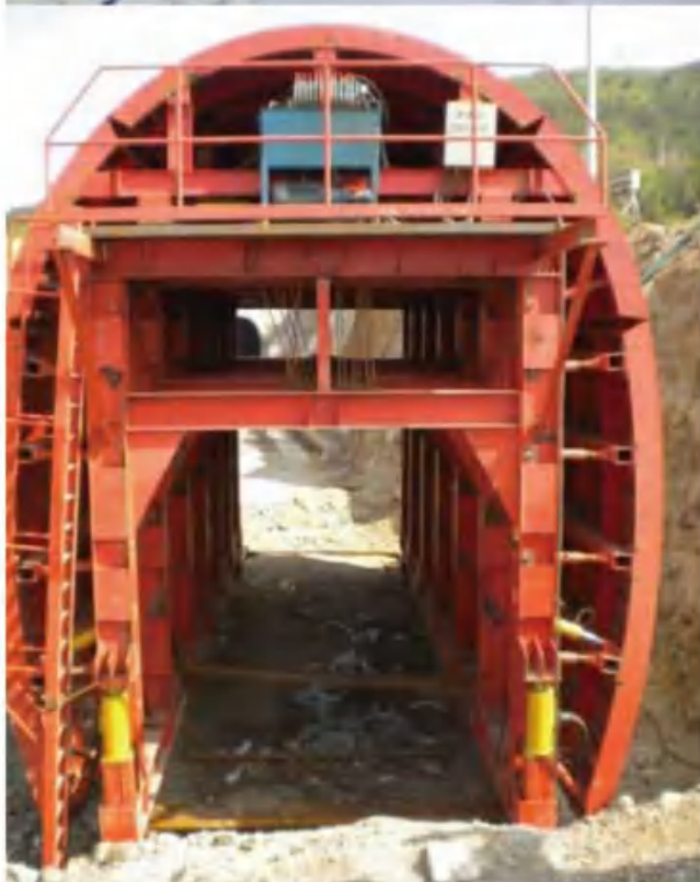
Project: Jinzhou—Chifeng railway User: China Hydropower 14nd Bureau Technical Data: length 12m; radii 2.5m; weight of trolley 70t Site photograph
