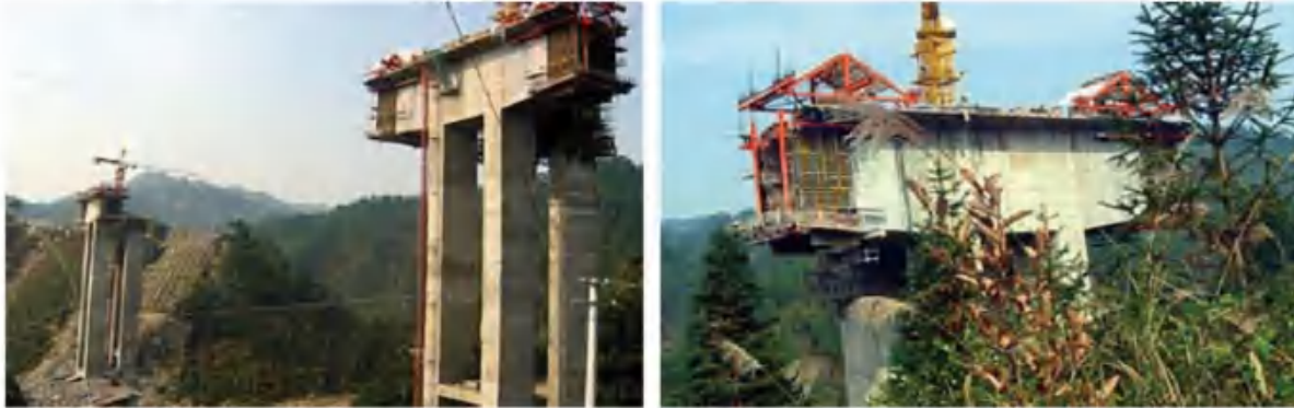
Guyed Traveler Formwork
