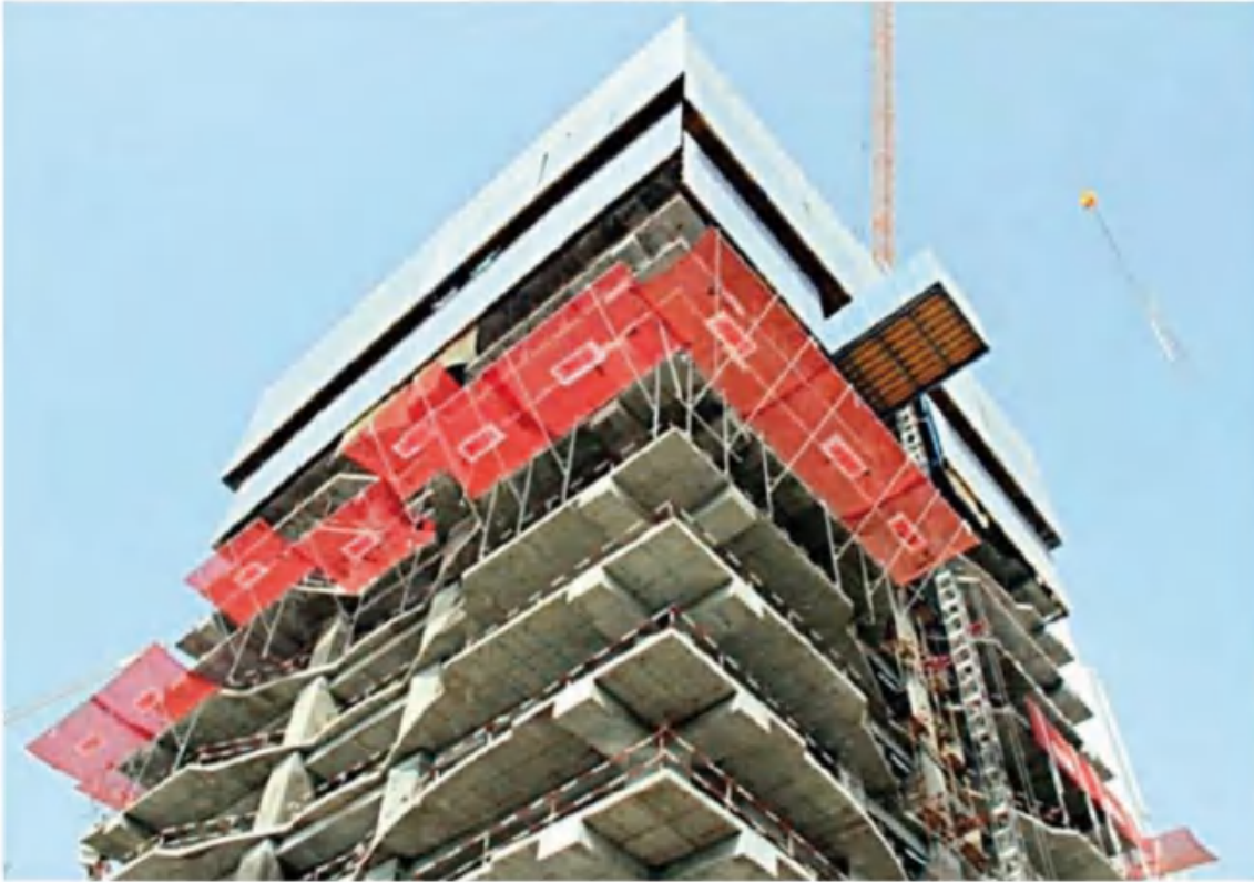
AL Hikma Tower, Dubai, UAE
