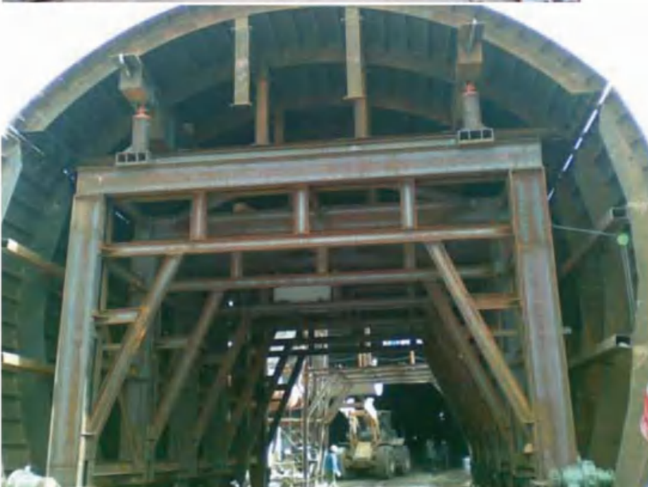
Project: Jinzhou— Chifeng railway User: China Hydropower 14nd Bureau Technical Data: length 12m; radii 4.34m; weight of trolley 105t Site photograph
