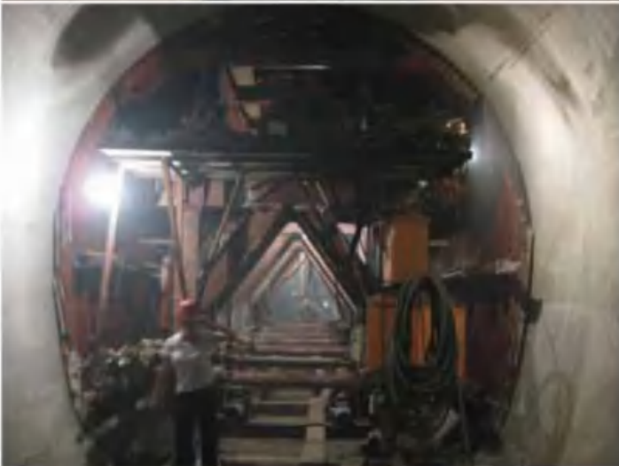
Project: Beijing Subway User: China Railway 2nd Bureau Technical Data: length 9m; radii 2.5m; weight of trolley 38t Site photograph
