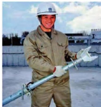
Assemble prop head and spring bolt
