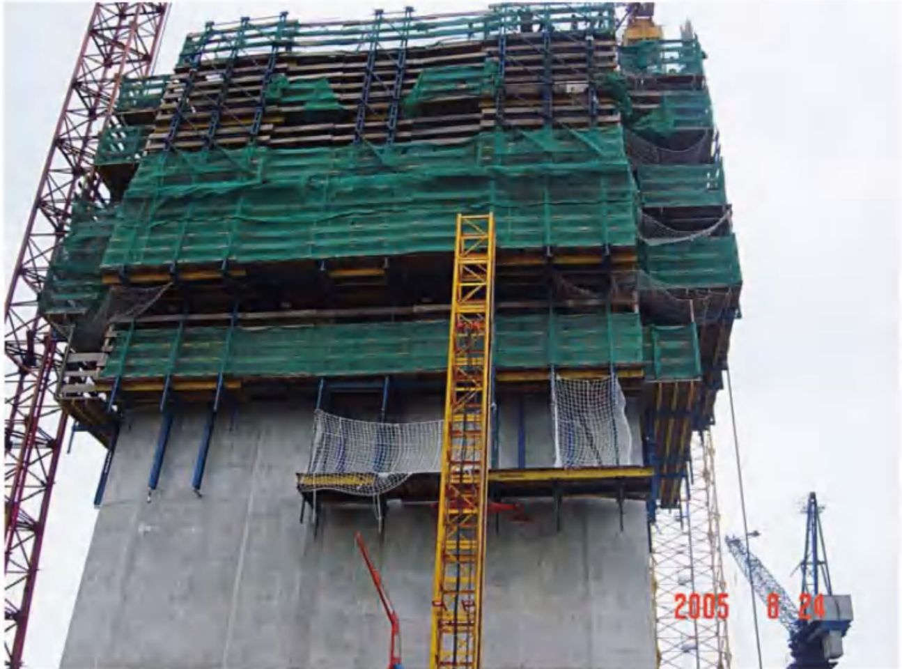
Sutong Bridge, Jiangsu, China
