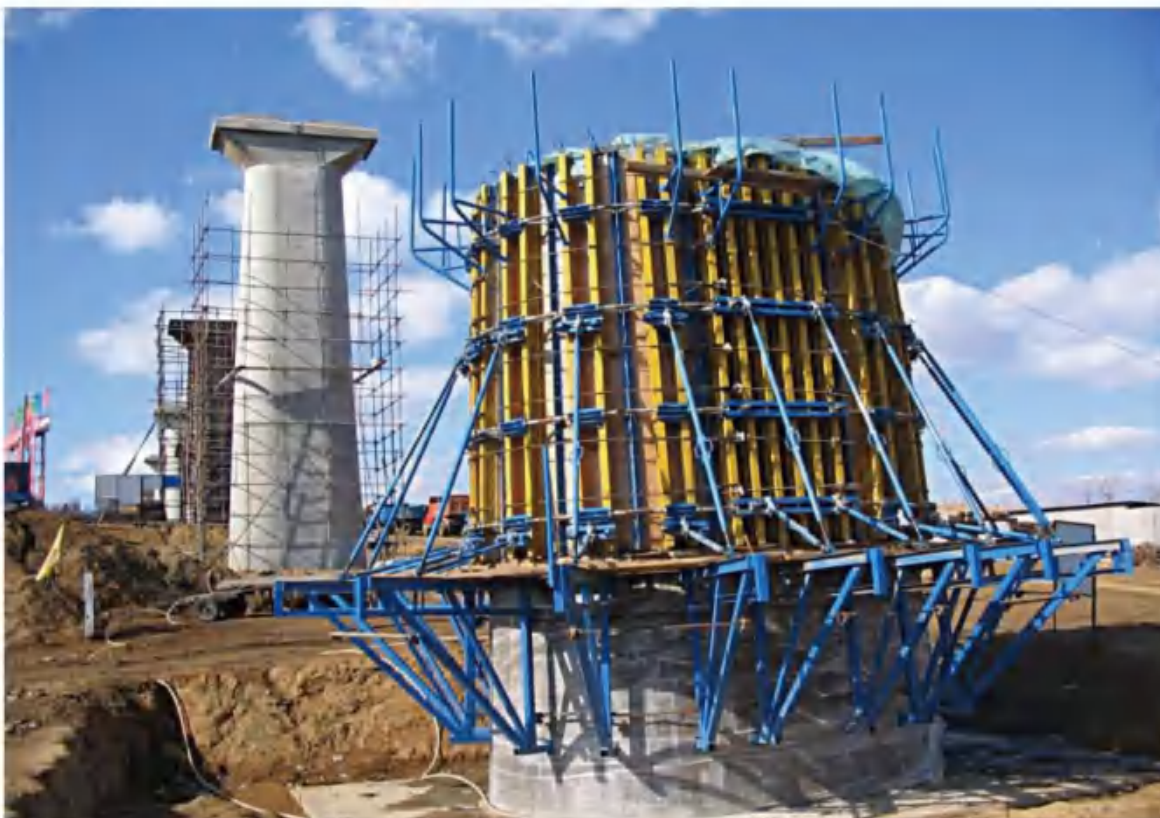
Nandaocun Bridge, China
