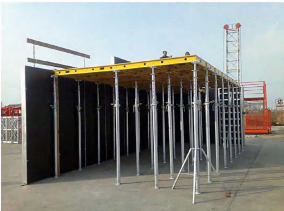
For Aluminum Frame Slab
